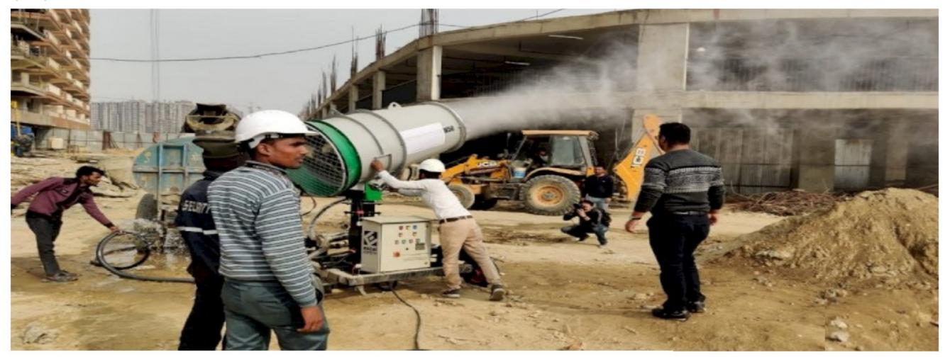
**Noida Extension**: Leading realty firm Gaurs Group has taken a major step to control the dust particle pollution at the construction sites. The company has installed a water gun at its project 7th Avenue, Greater Noida West, that will help settle the dust. The decision -- a first not only in Delhi NCR but whole of North India -- was taken after rising concerns that construction sites are adding to the environment pollution.
