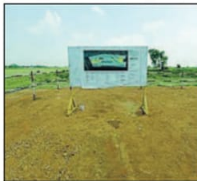
Jewar airport construction site in Greater Noida. HT ARCHIVE
